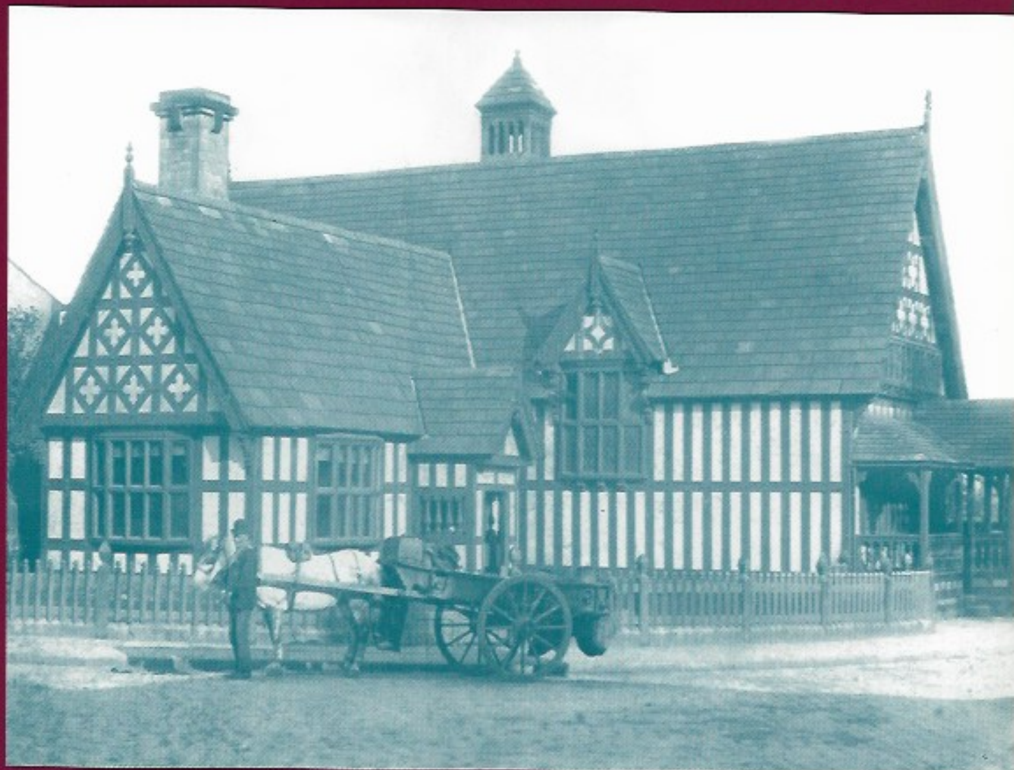
Worsley CourtHouse as originally built c1890
